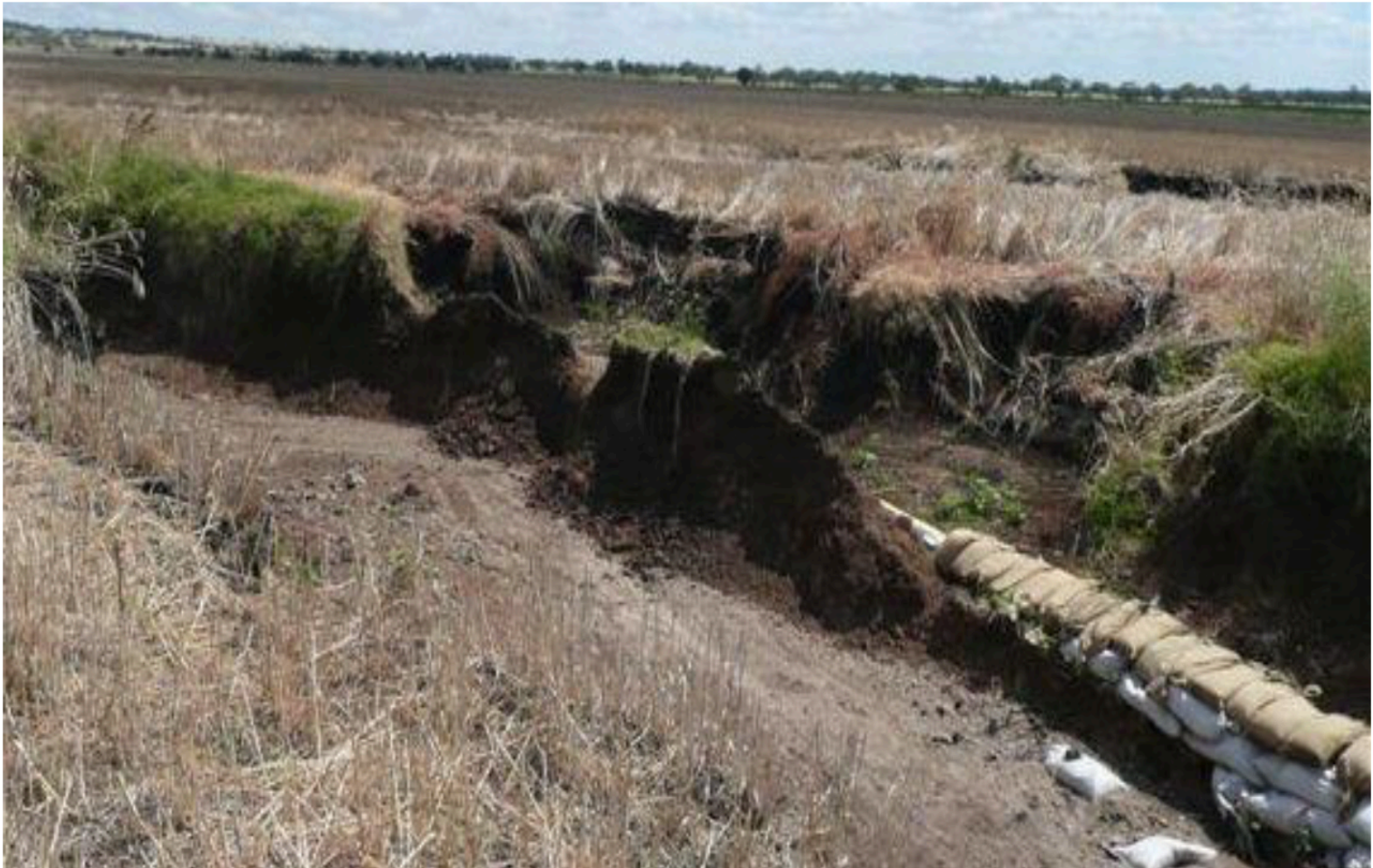
Photo 1: Gully and exposed pipe at Berana with spur gully following pipeline
