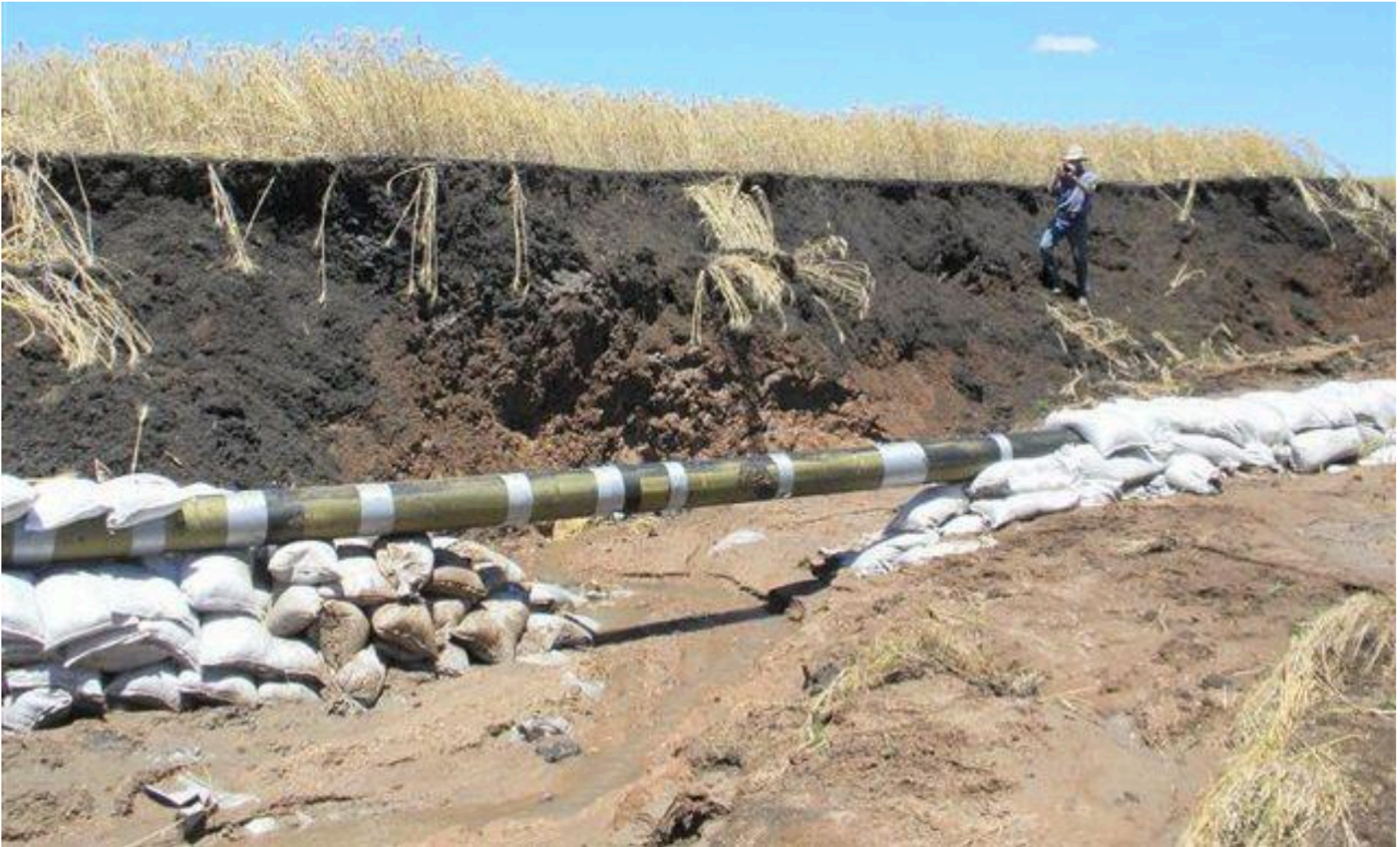
Photo 2: Gully and exposed pipe at Berana with failed sand bag supports
